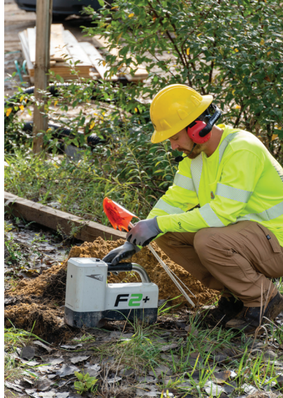
PICTURED: (Above) River Gauthier, Outside Plant Equipment Operator, running the boring machine. (Right) Josh Bergakker, Cable Splicer, working at the pedestal as Acentek hooks up a new home in Allendale to fiber optics.
