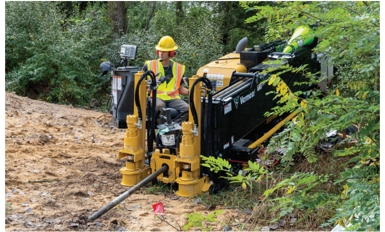
PICTURED: (Above) River Gauthier, Outside Plant Equipment Operator, running the boring machine. (Right) Josh Bergakker, Cable Splicer, working at the pedestal as Acentek hooks up a new home in Allendale to fiber optics.
