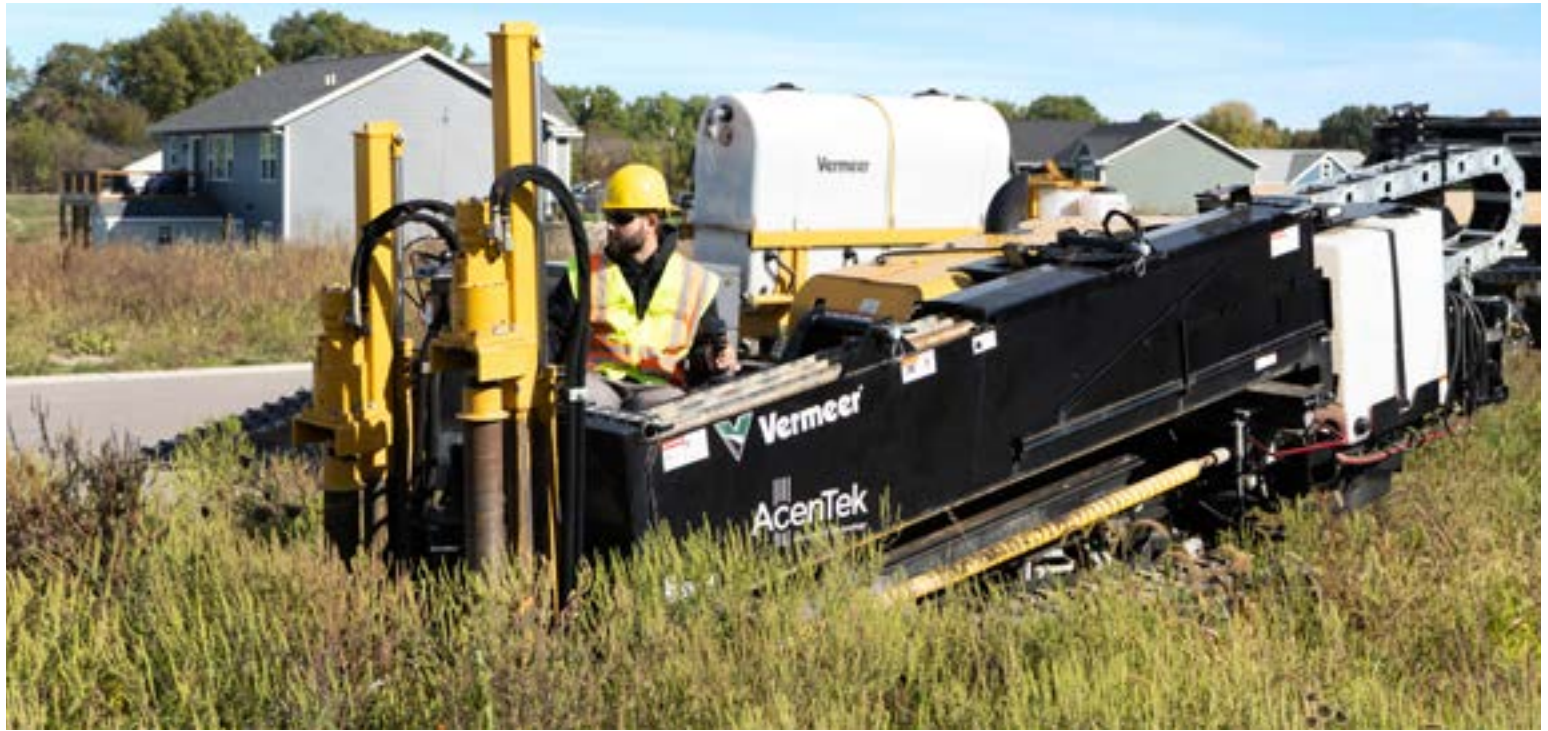
Outside Plant Equipment Operator, Hunter, runs a boring machine to prepare for fiber insertion.
