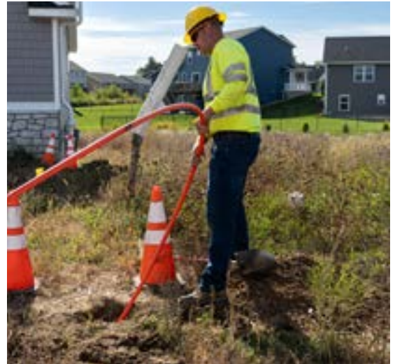
Josh Bergakker, our Outside Plant Coordinator/Splicer pulls duct work where fiber will be inserted.
