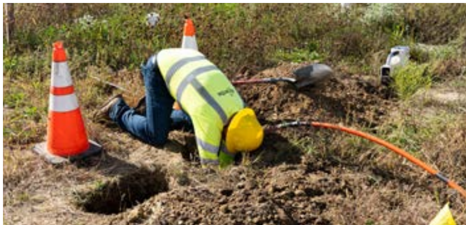
Josh prepares the hole for connecting the duct work.
