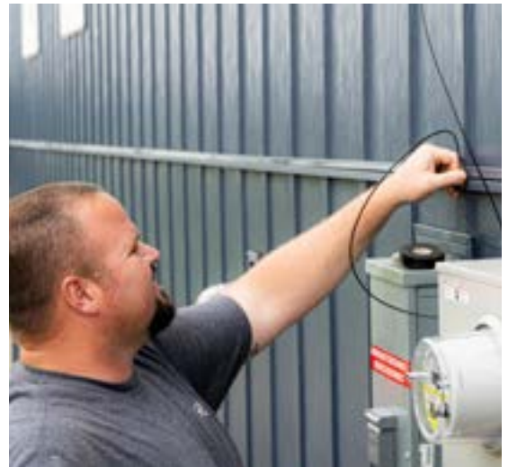
Combination Tech, Ron Aten, prepares to hook up a home to fiber by connecting it through the box on the exterior of the home.
